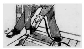
Temporarily support the floor area to be worked on, ONLY if intending to replace more than one joist end at a time. Cut back decayed joist end(s) as far as necessary to reach sound timber.
