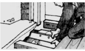
3. Place the two 'L' sections of the Sovereign Bower Beam unit one each side of the joist, then slide the nearest ends a minimum of 110mm (4") into the joist socket. Position the two sections of the resulting U-Beam in place, by hammering in the galvanised locating pins, through the SMALL holes, (but NOT opposite each other, to avoid clashing).
