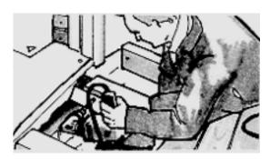
4. Using the LARGE holes as a guide, drill the appropriate NUMBER of pilot-holes in the joist, but again, NOT opposite each other. Use a 5mm (3/16") bit, to a depth of 30mm (11/4"). For 'numbers', first refer to FIXINGS on previous page. (Hardwood joists will require deeper holes - please consult our Technical Department).
